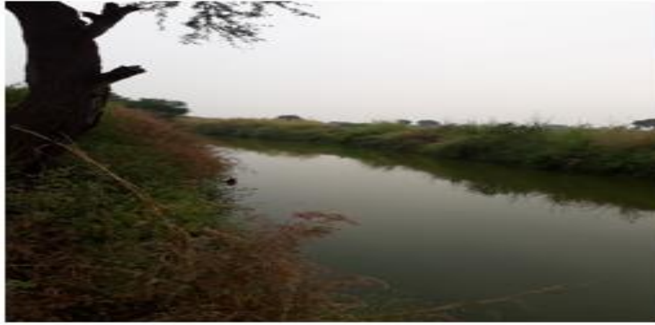
Nala Deepening and Widening
